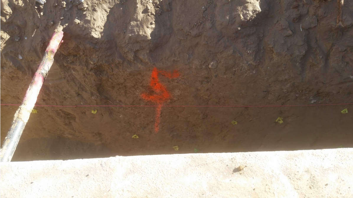
FT-4 Southern trench wall, Station 0 + 05'
