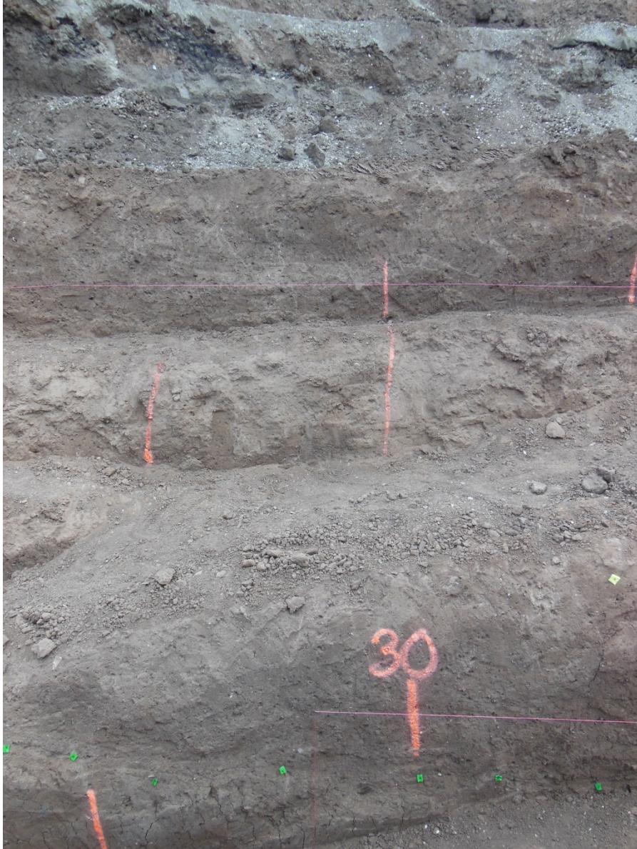
FT-3: Southern trench wall, Station 0 + 30'
