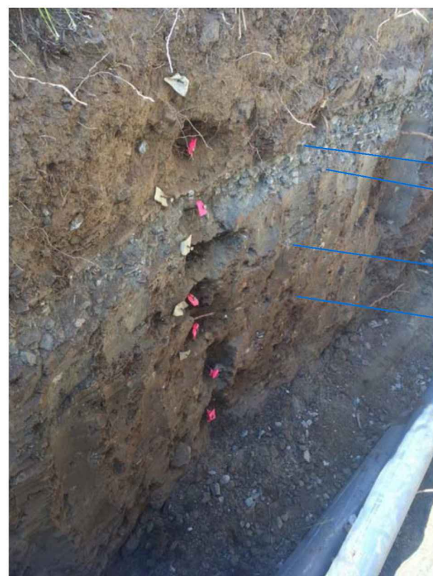
Stratigraphy and sample locations (pink flags) on the south wall of the Wilshire Boulevard Utility Trench. View to the southwest. Blue lines show the approximate location of contacts denoted on the geologic log to the right of photo.
